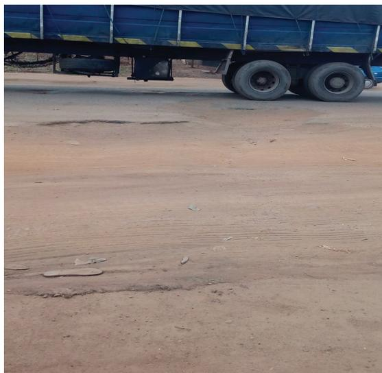
Figure 2: A failed section of the road exposing the roads foundation and relatively thin asphalt riding surface.
