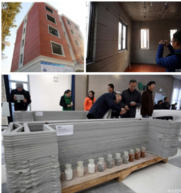
Figure 7: 3D printed buildings in China during 2014-2015.
