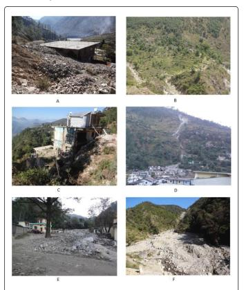
**Figure 8:** Heavy localized rainfall/cloudburst induced debris flows through the streams; (a) newly constructed house filled with debris at Siligi tok (Lingari Gramsabha); (b) agricultural land damaged at Bansoli village; (c) severely damaged house just below road at Sunali village; (d) damaged structures at Ghat; (e) partially damaged Tefna village; (f) washed off road section lead to Ghat-Bhenti.
