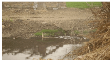
Figure 9: Pipes dumping wastes from houses into Mariotteya water stream.
