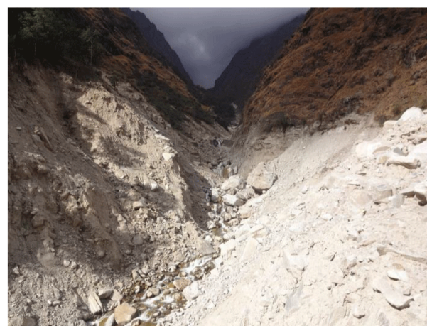
Figure 12: Upstream side view of Malpa Gad.
