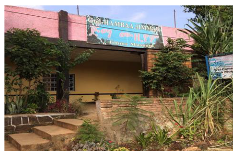
Figure 9A: Partial view of Jimma museum from main gate.
