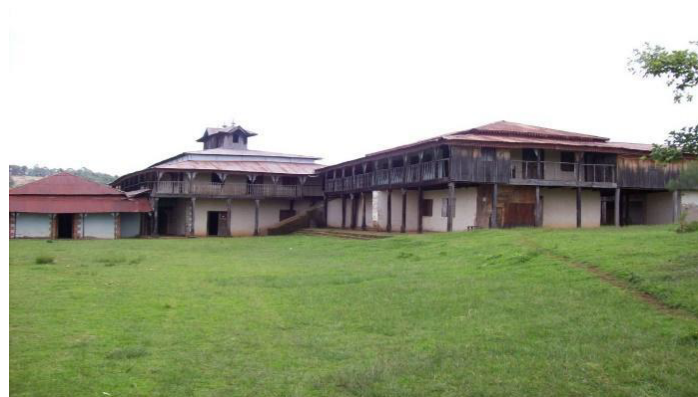
Figure 6A: Partial view of Aba jifar palace from the west.
