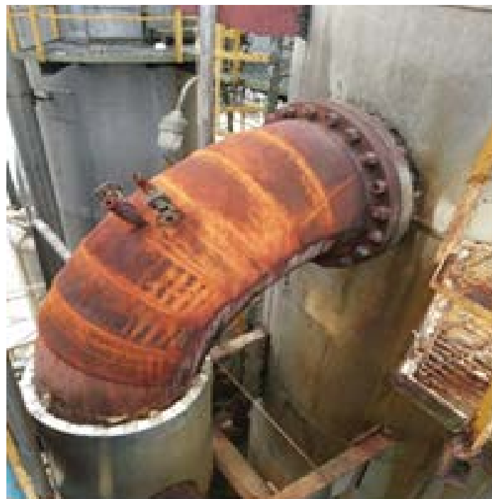
Figure 1: Welding photo of elbow.
