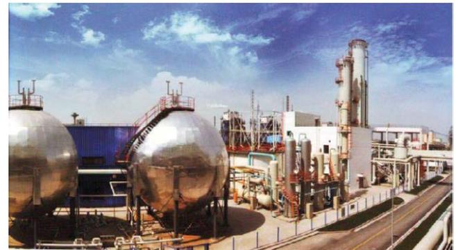
Figure 1: 120,000 t/a Post-combustion capture from coal-fired power plant in Shanghai.
