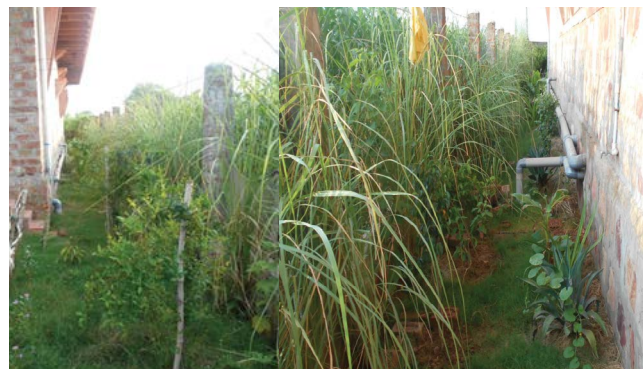
Figure 7: Waste water treatment at individual level (RSNH Centre, Rajputana's Shakuntalam, Village Ramnagar, Bharatpur, Rajasthan, India).
