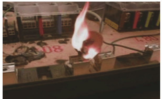
Figure 1: Showing catastrophic failure of Metal Oxide Varistor during tests, Source: Brown, 2013.
