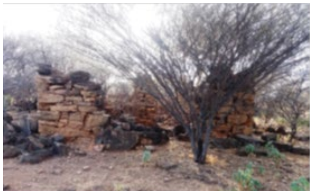
Figure 1: Ruined stone built house at derbi belanbel.
