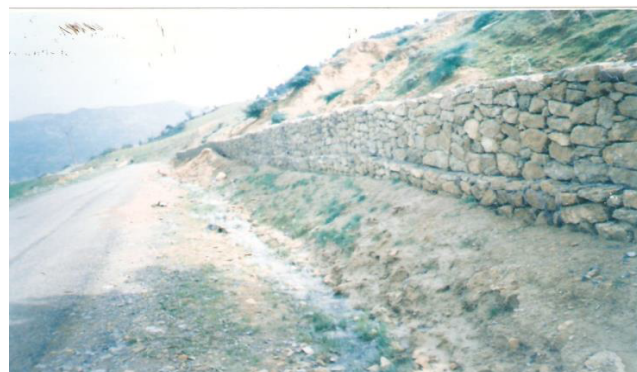
Figure 7: Natural drainage ditch along the road.
