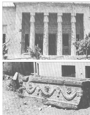
Figure 4: Beirut National Museum devastated by bullets and shells in 1991, and a broken Roman sarcophagus outside the wrecked Museum.
