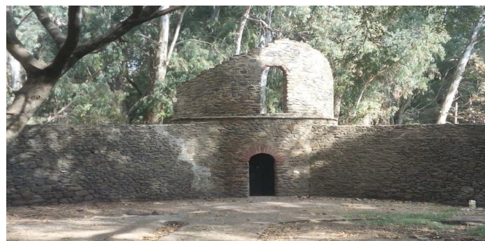
Figure 14: The guard house found on the south of the bath.
