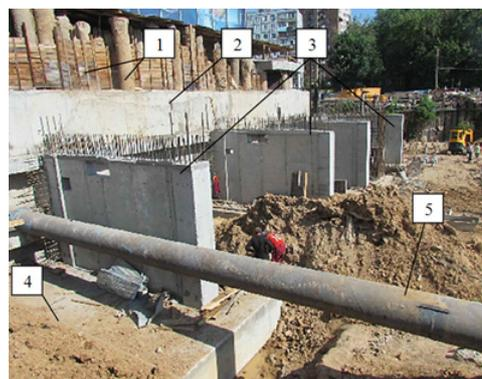
**Figure 2:** Fragments of cast in-situ reinforced concrete buttresses: 1-existing boring piles of pit fencing; 2-fencing of cast in-situ reinforced concrete; 3-monolithic reinforced concrete buttresses to reinforce the existing retaining wall; 4-monolithic reinforced concrete grillage; 5-existing gain firing pipe.
