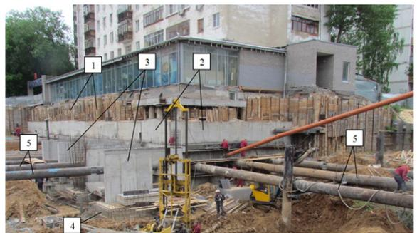
**Figure 1:** The scheme of retaining walls of the boiler is fixed by 1000 mm steel tubes: 1-existing boring piles of the pit fence; 2-fencing of cast in-situ reinforced concrete; 3-monolithic reinforced concrete buttresses to reinforce the existing retaining wall; 4-cast-in-situ reinforced concrete grillage; 5-existing steel tubes for reinforcing retaining walls.
