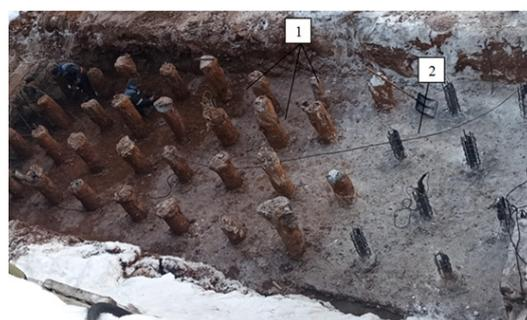
**Figure 3:** Pile field under monolithic reinforced concrete buttress: 1-heads of injection EDT piles; 2-concrete preparation for the construction.
