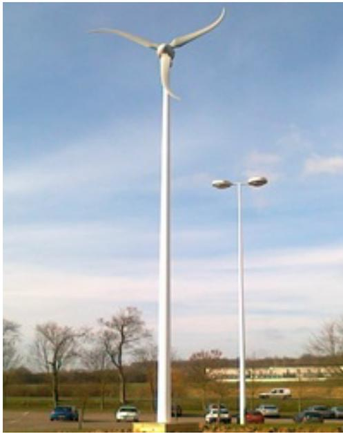
Figure 2: The 3 blades wind power skystream of the GREEN platform.
