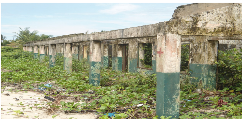
Figure 16(a): Former Itak Abasi Health Center damaged by the storm surge in 2011.
