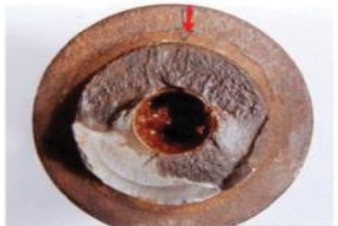
Figure 3: crack initiation site is marked red.
