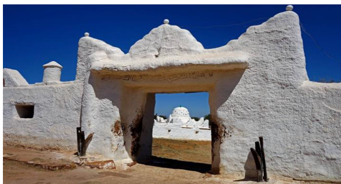
Figure 2: Partial view of the site from the west or main gate.
