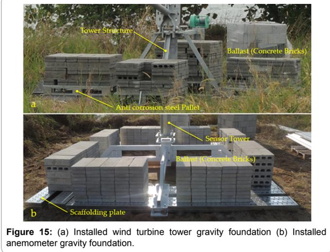
Figure 15: (a) Installed wind turbine tower gravity foundation (b) Installed anemometer gravity foundation.
