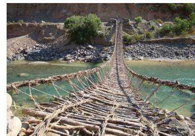
Figure 3: Tinkuychaka, a suspension bridge over the Pampas River, Central Peru.
