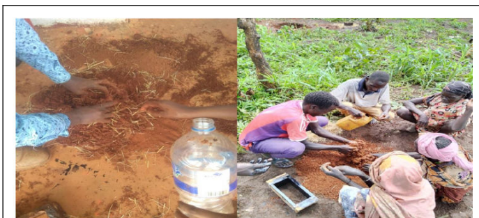
Figure 5: Mixing the soil and the straw at the site and mixing the soil and the straw with water the site.
