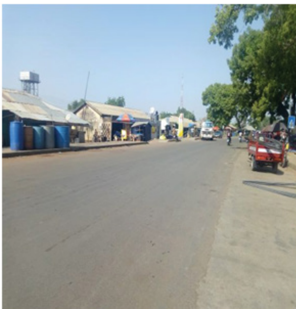
Figure 7: Damongo-Sawla road (Source: Field survey, 2020).
