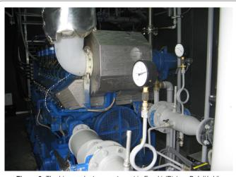
Figure 6: The biogas plant generator set in Franki (Picture B. Igliński).
