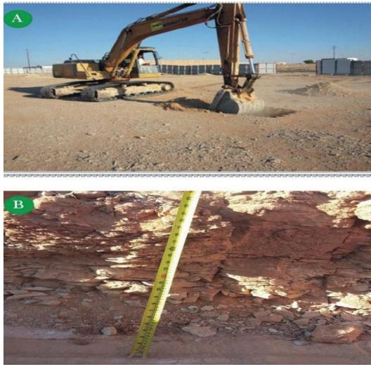
Figure 4: A- the JCB drilling the test bit, B- the depth of test bit.
