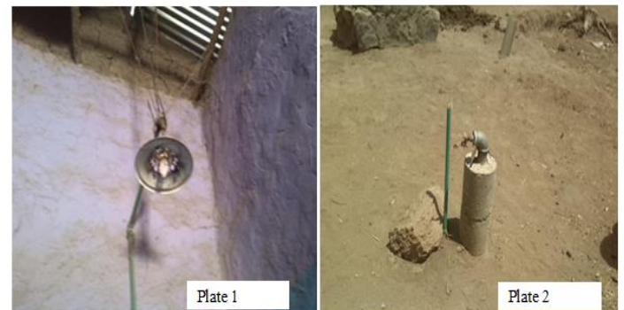
Figure 3: biogas plant that has been abandoned due to lack of maintenance. Source: Photo taken during field observation.
