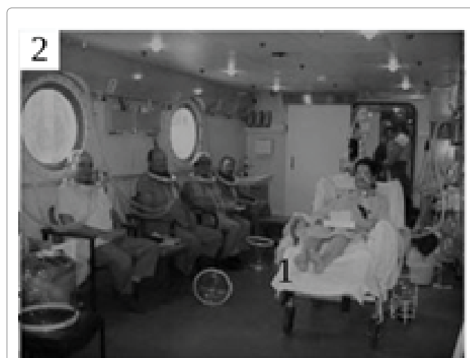
Figure 2: Clinical multiplace hyperbaric oxygen chamber (Courtesy of Fink Engineering, Warana, Queensland, Australia).
