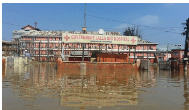
Figure 13: Tertiary care Lalla Ded Maternity Hospital, Srinagar (inundated)
