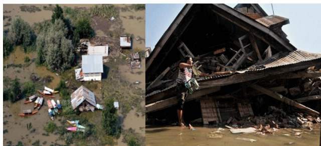
Figure 7: Shattered dreams and debris of the houses
