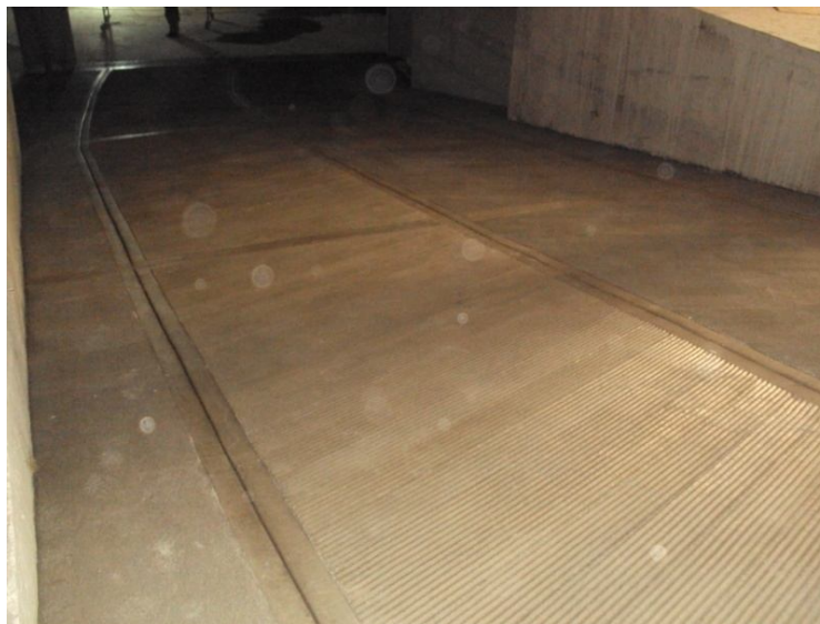
Figure 2.1.1: Ramp of Underground Parking
