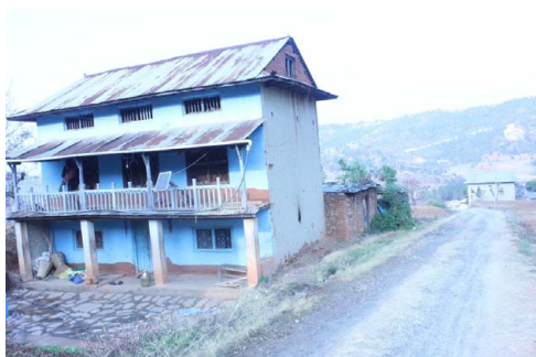
Figure 16: A road approaches towards preserved and renovated statue of Guru Jambheshwara Ji. From this place, it is in South Eastern direction, nearly 50 Meters [4].
