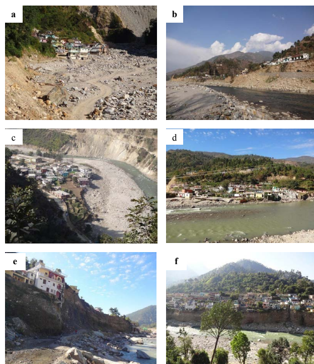
Figure 4: Deluge of June, 2013 events caused devastation in these towns; (a) Sonprayag, (b) Chandrapuri (c) Tilaknagar, (d) Ganganagar, (e) Vijaynagar, (f) Tilwara. All these towns situated over river borne materials (RBM) terraces along the banks of Mandakini river.
