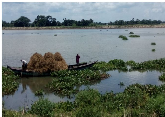
Figure 3: Pictorial view of Dhonagoda River and its embankment.
