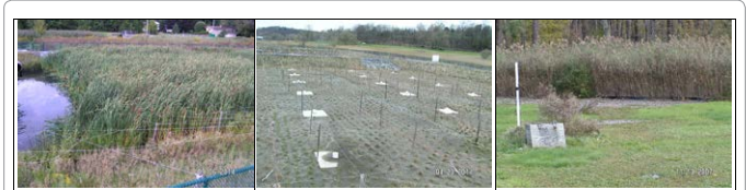
Figure 1: Appearance of full-scale constructed wetlands: a FWS wetland with well-established vegetation (left), a newly planted VF wetland with risers on concrete distribution pads (middle), and a HSSF wetland with planted and unplanted zones (right).
