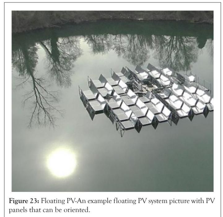
Figure 23: Floating PV-An example floating PV system picture with PV panels that can be oriented.
