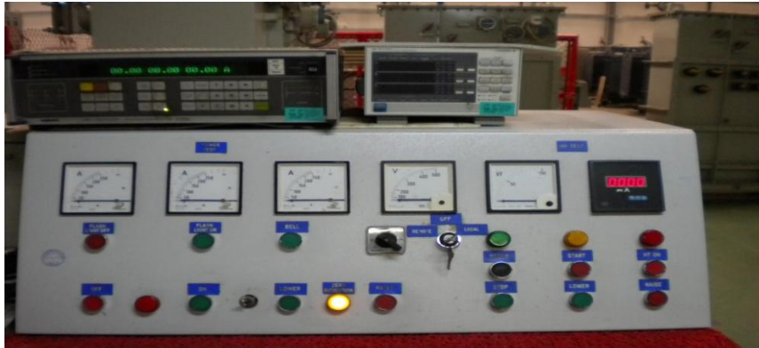
Fig 5 : No Load Loss Control Panel
