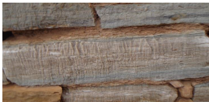
Figure 8: This is one of the longest of the marble stones, which the masons significantly used to construct the Mosque. The stone slab measures about 1.3 meters long. The lime mortar firmly bounded the stones.
