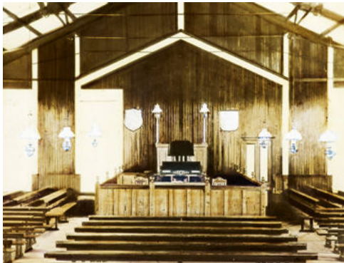
Figure 3b: The interior view of the church.
